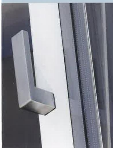
Top: detail of hinged patio door with tilting window; has a multi-point lock with connecting cylinder. Left: casement window without plate with handle fixed directly onto glass
